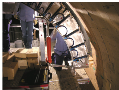
FDEF adjusts easily in less than 10 minutes inside the kiln
